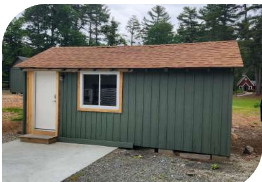
Door & Window replacement at Mill Street Recreation Snack Shack
