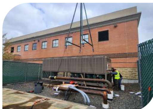
Replacement of two 200-ton chiller units at the Ahern Middle School
